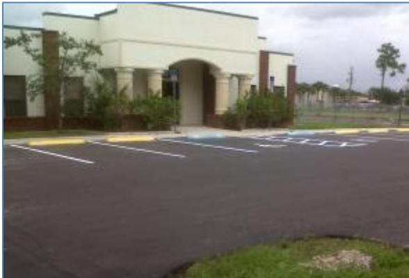
The finished concrete parking lot with asphalt atop geotextile fabric will enjoy a longer life and greater value than traditional asphalt applications.
